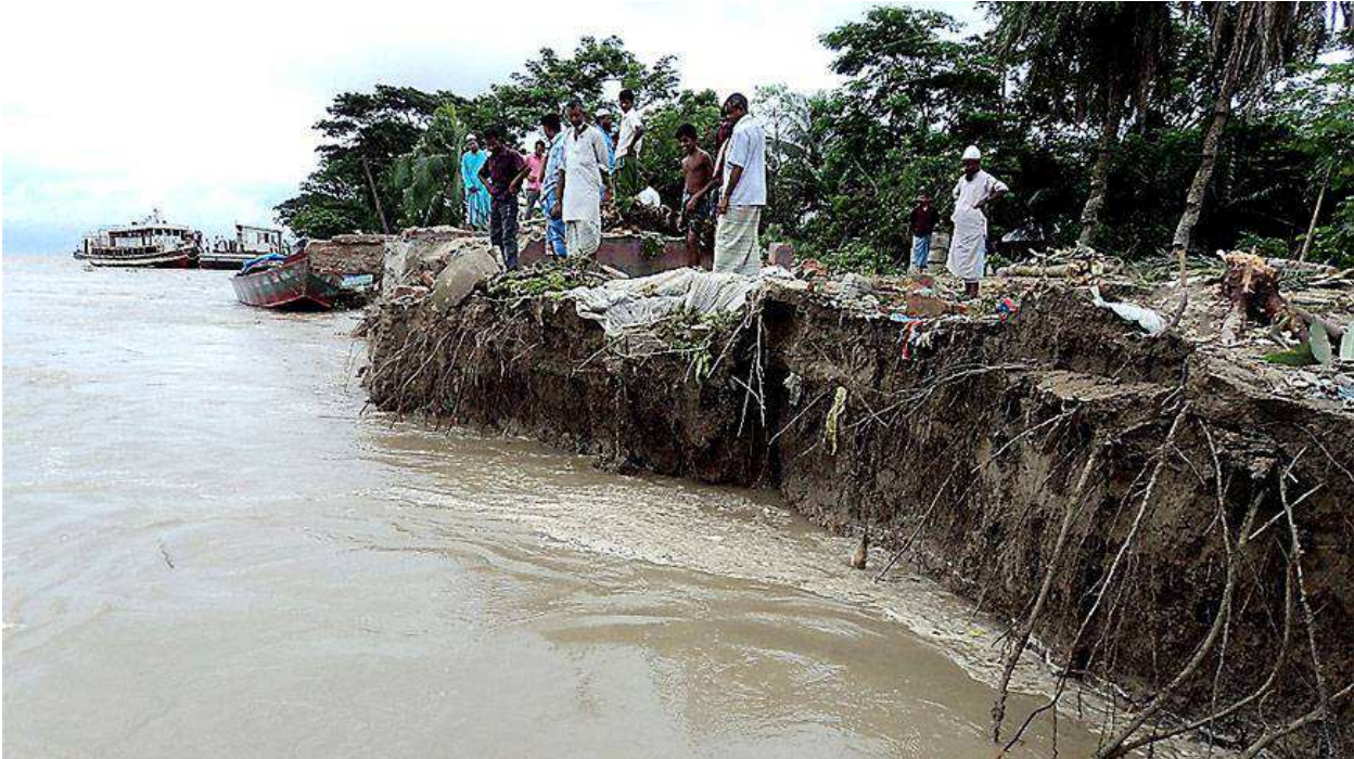
Eroded bank of the River Jamuna
